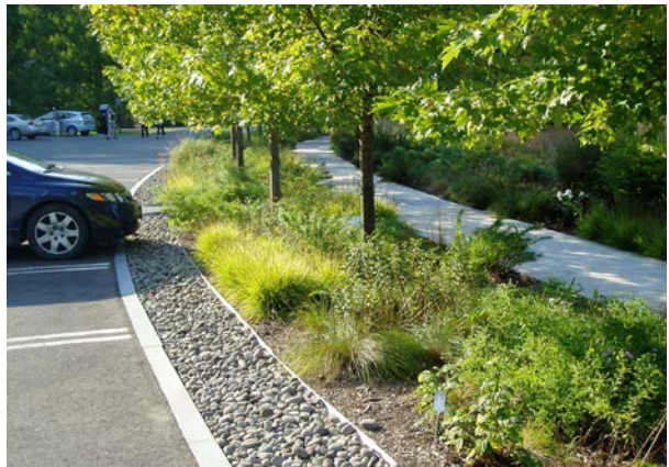
A parking lot utilizing Low Impact Design (LID) strategies, including permeable paving, a stone infiltration strip, and a bioswale.
