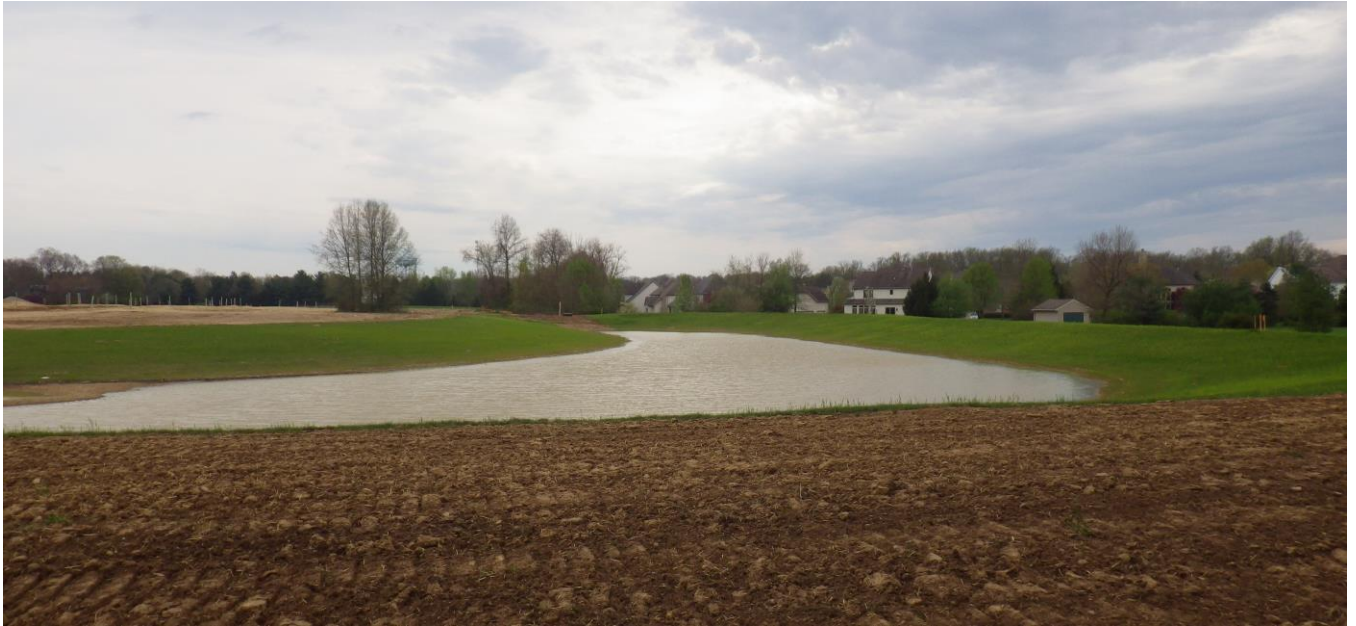
Figure 12: Proper sediment basin stabilization
