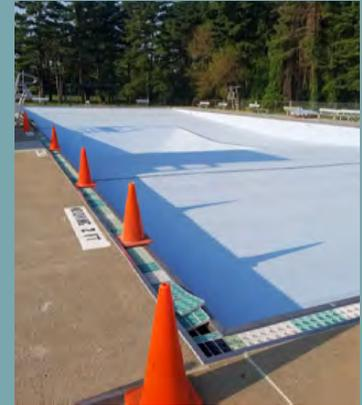
**Front Pool Liner** – The installation of the liner in the front pool of the Gahanna Swimming Pool provided a resourceful option to ensure the safe and effective operation of the facility for future years.
